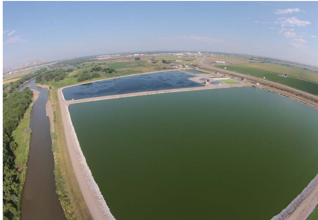
City of Scottsbluff, Wastewater Treatment Plant
