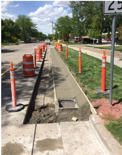
18th Street & 3rd Avenue
